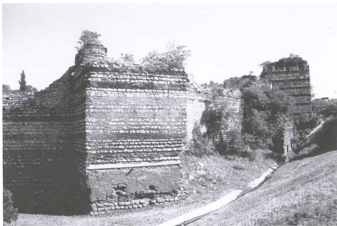
Plate 56 Wall of Manuel I Komnenos
